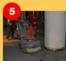
5 Polishing the floor in several cycles using planet grinders with TERRASEAL
