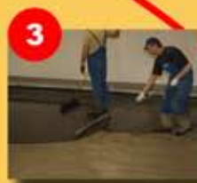
3 Spreading 15-30 mm thick layer of TERRATOP
