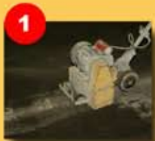
1 Preparation of concrete base
