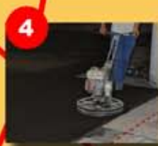
4 Trowelling with a power trowel for complete closure of porosity
