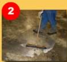
2 Priming with BAUBOND and BAUGRUNT
